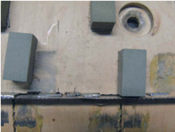
Shimming of the lead edge is a clear indicator failure is imminent.
